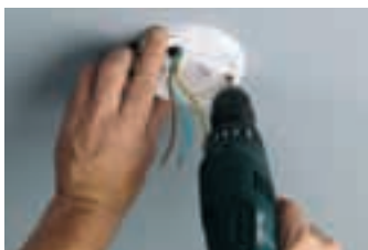
Fix the centre plate in place.
