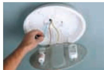
Connect the wires to the connectors.
